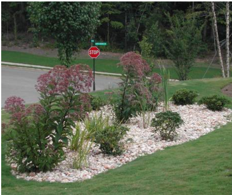
Bioretention area in The Estates at Brooke Park, Canton. Photo courtesy of Diane Minick.
